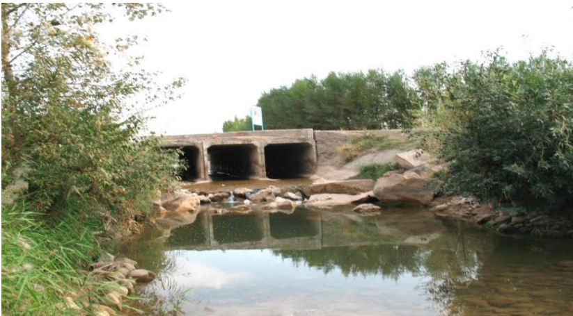
Figure 9. Bridge crossing (PC 88+83)
