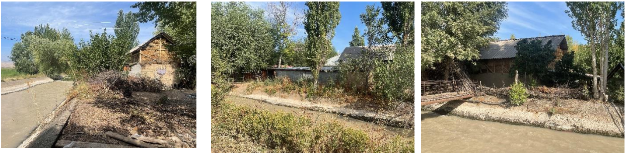
Figure 17. Buildings near MC Levaya Vetka from PK39+00 to PK50+00
