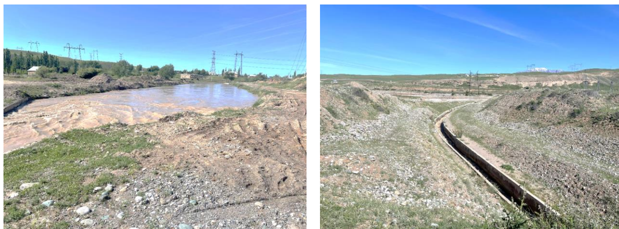
Figure 4. Single chamber settling tank with discharge channel
