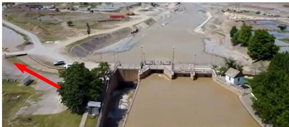
Figure 3. Main water intake structure
