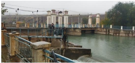
Image 4. Head water intake structure
